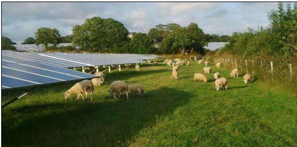
Figure 8.4: Ground Coverage Under Arrays – Example 1
